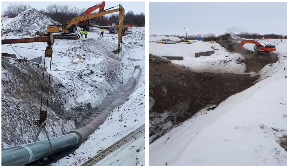
805 + 720 Track hoes backfilling open ditch at the Pipestone
