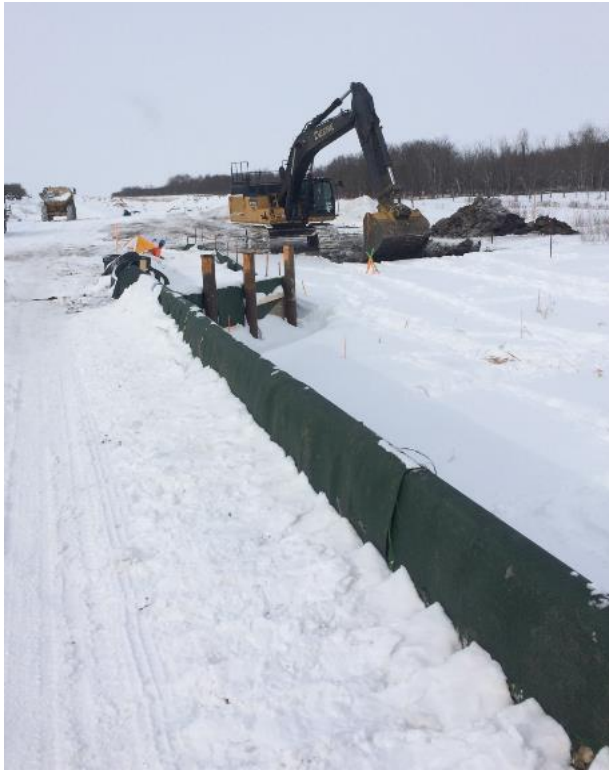
Stony Creek SK WC 89 Excavating ditch line, placing WC material on geo & sand shading pipe.
