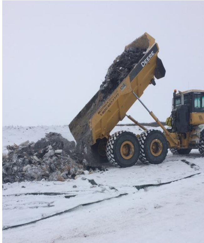
Stony Creek SK WC 89 Excavating ditch line, placing WC material on geo & sand shading pipe.
