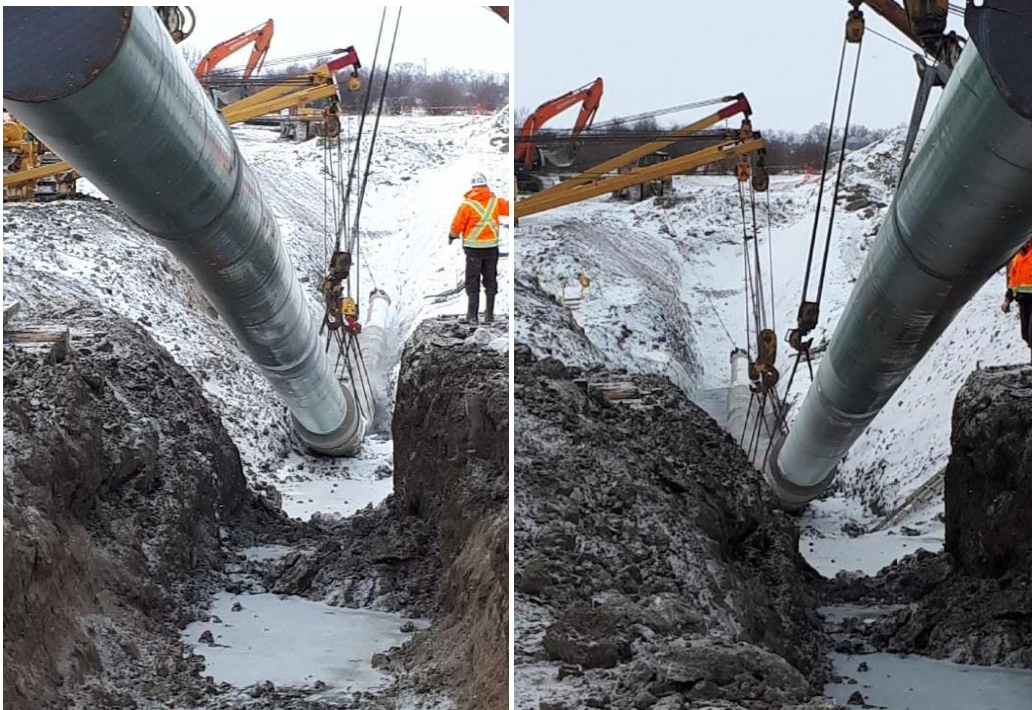
805 + 700 Lowering pipe across the Pipestone Creek MB 1010
